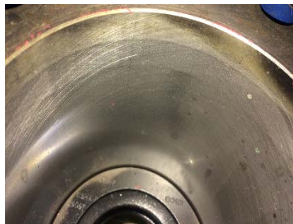
Figure 1b: Damaged sleeve
